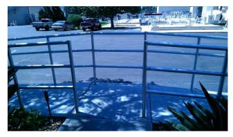
maneuverability. The width of ramp must be at least 48" wide. The handrail must have 12" extensions at each termination. The ramp must have a guide curb on the surface that must be a minimum of 2" high. The entry ramp is deficient in all of these areas.
