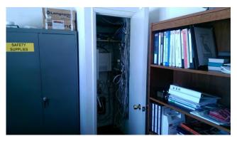
Egress from the office must egress directly into a corridor or outside to meet exiting requirements. The adjacent control room and the adjacent workstation are considered intervening rooms. The current path egress from this room may be considered a life and safety hazard.
