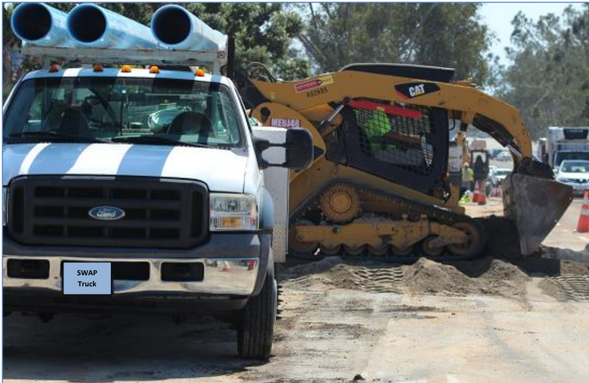
The City of Del Mar's Sewer, Water, Arterial, Paving ("SWAP") Project
