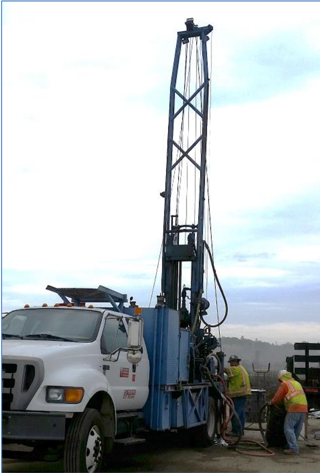
Geotechnical sampling for land outfall replacement
