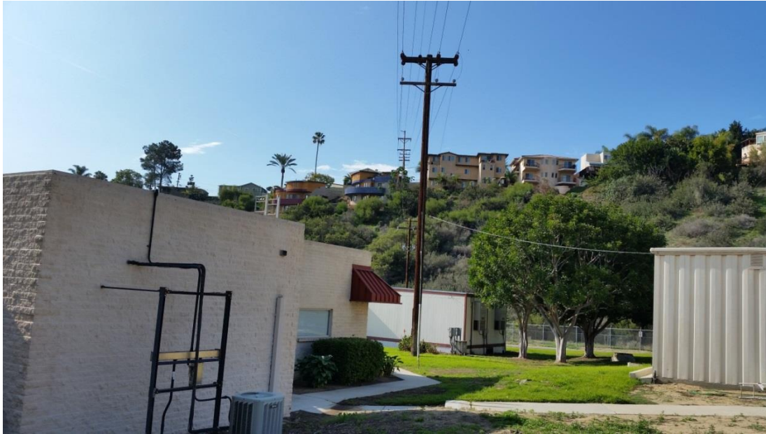
Photo 2 Buildings under power lines
