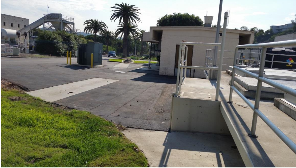
Photo 1 Maintenance-Rated Guardrails at Treatment Facilities
