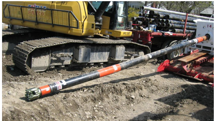
A mud motor and bit is shown here for soft soils.
