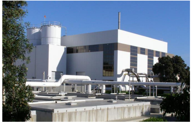
Shown here is the completed Encina Phase V Expansion Biosolids Building. Eric Sturtz served as the Construction Manager for this award winning project.
